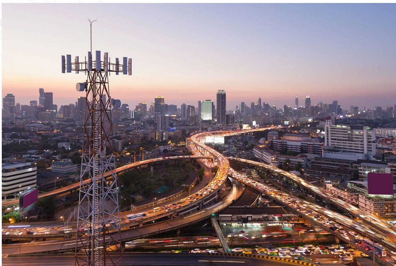
Figure 1: tower with 5G cellular network antenna on city background
