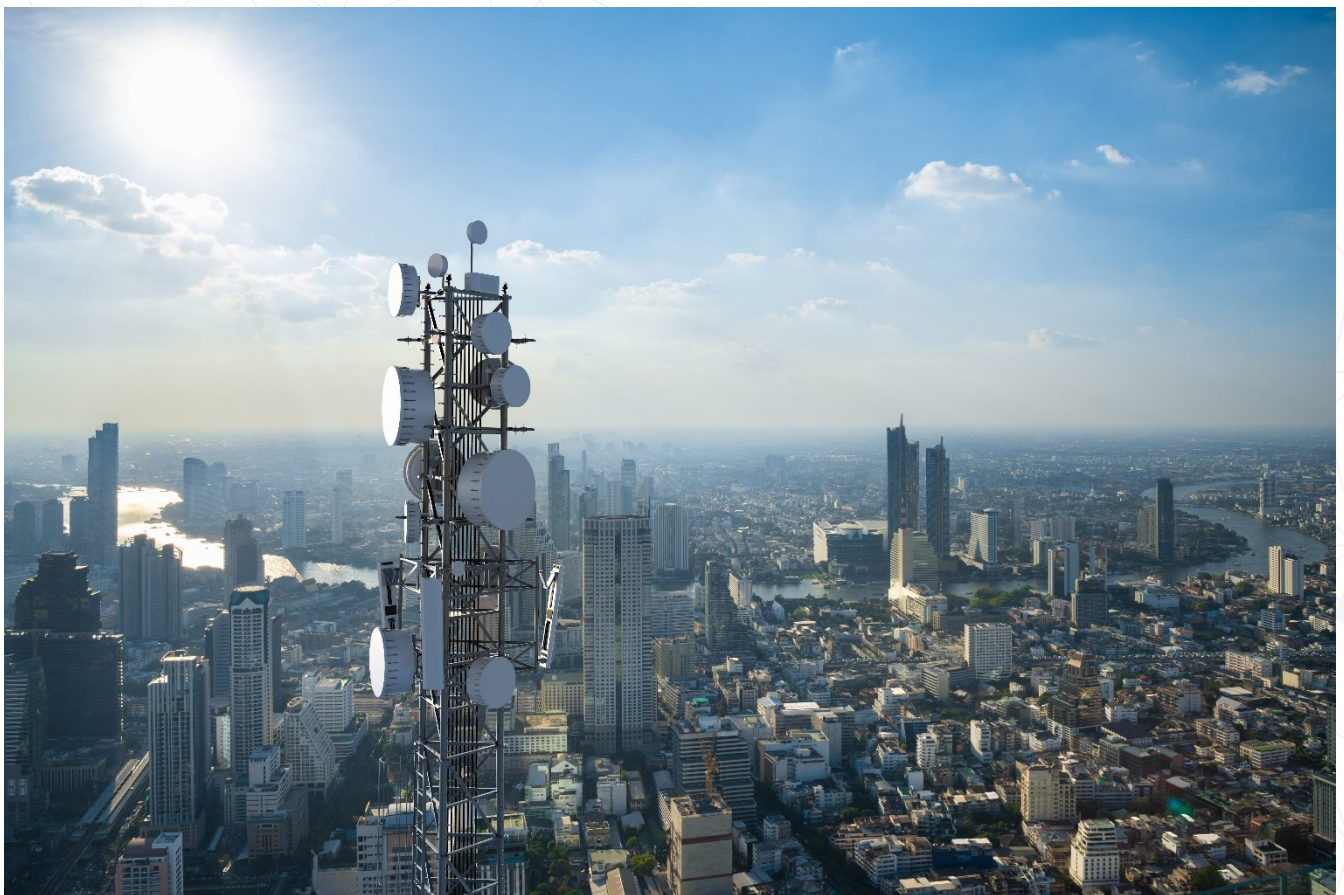
Figure 2: Telecommunication tower with 5G cellular network antenna on city background
